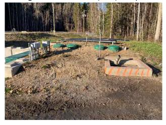
L) balancing tank. Lift station #3's level is controlled by an ultrasonic transducer inside the lift station and is monitored by a PLC inside the MCC room. The wastewater from LS#3 is pumped into the aerated septage receiving lagoon for primary treatment.
